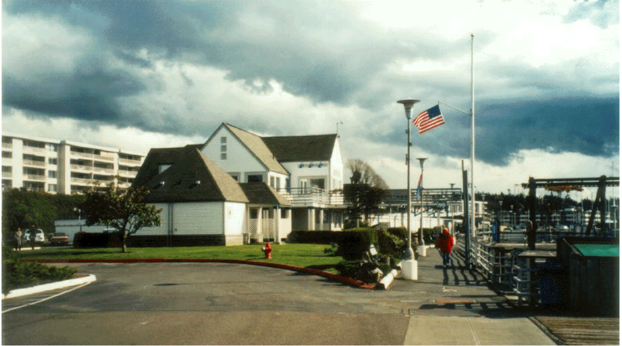
Figure 6-1. Marina Office Building
