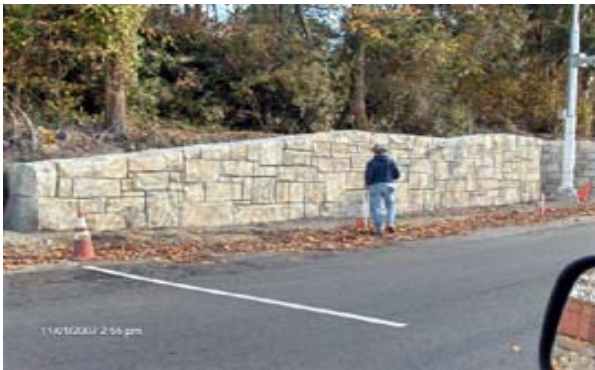
Retaining Wall near S. 260th St. (11.01.07)
