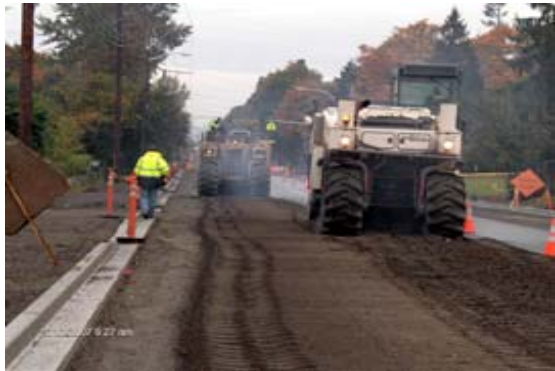
16th Avenue S. Paving Preparation (10.16.07)
