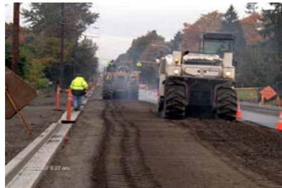
16th Avenue S. Paving Preparation (10.16.07)
