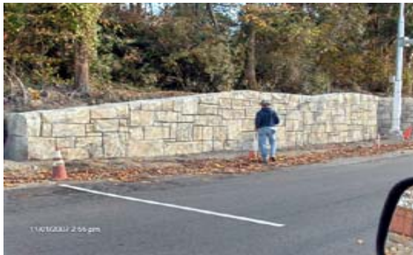
Retaining Wall near S. 260th St. (11.01.07)
