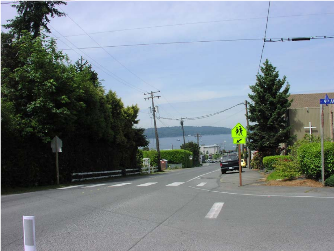
S 223 rd Street & 9 th Avenue S – existing conditions
