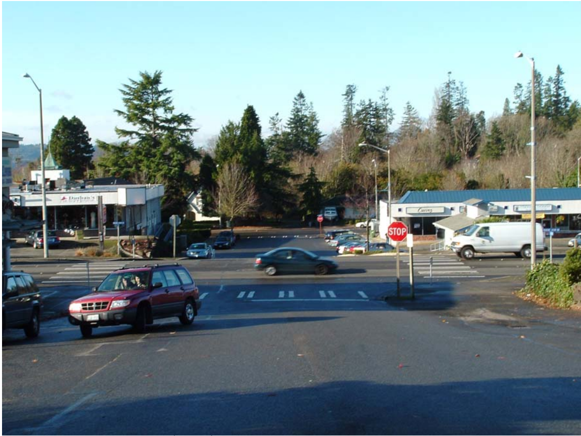
S 219 th & 8 th Avenue Alley – existing conditions
