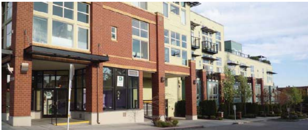
This parking structure contains usable office and retail space on the ground floor.
